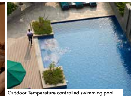
Outdoor Temperature controlled swimming pool
